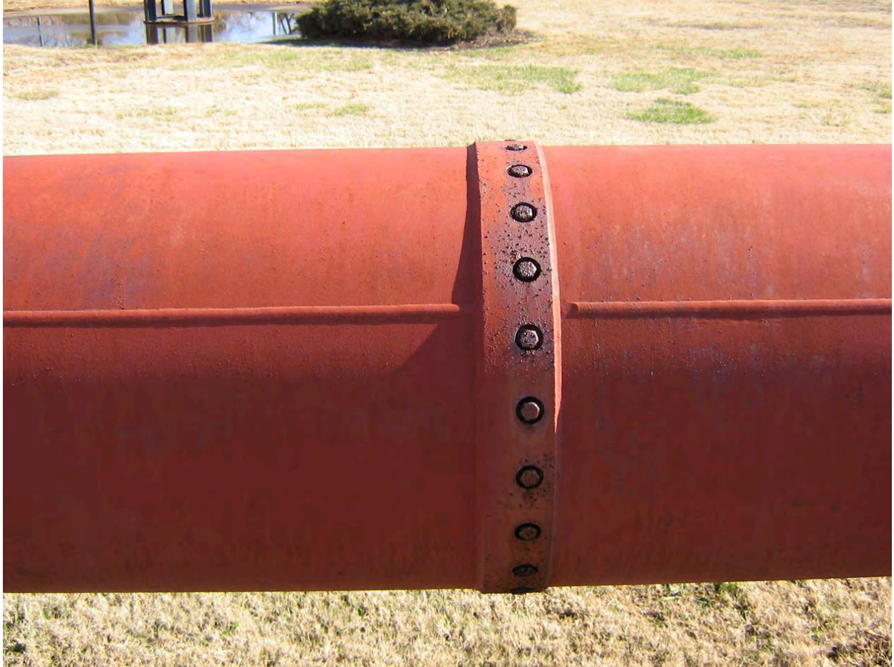
Photo 12: Bolted Mid-Case Band
