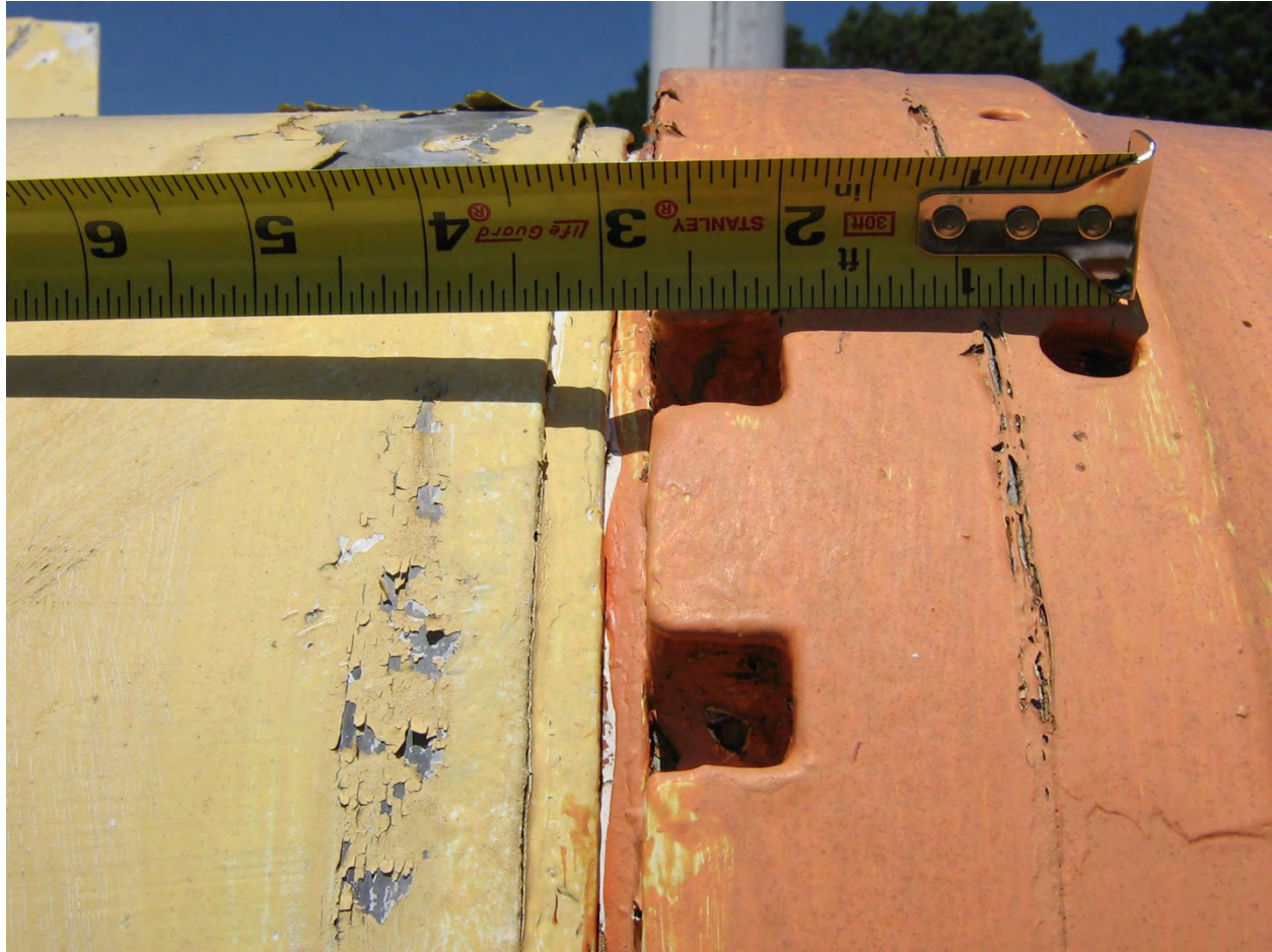
Photo 2: Nike Adapter Mounting Bolt Access Slots
